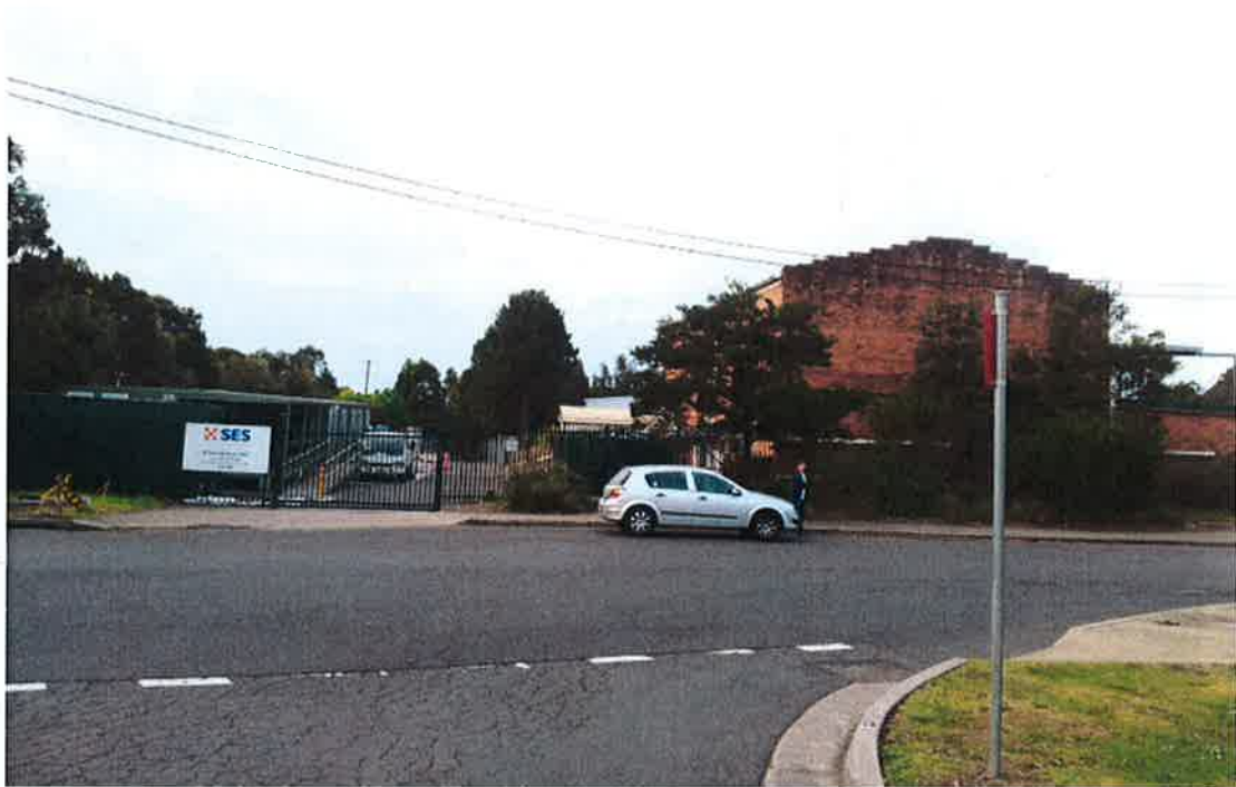
Photograph 7 – SES Depot, northern side of Weeroona Road.
